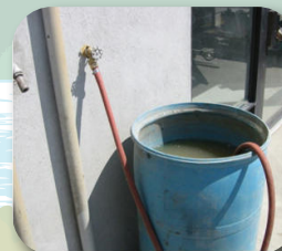
Improper connection
